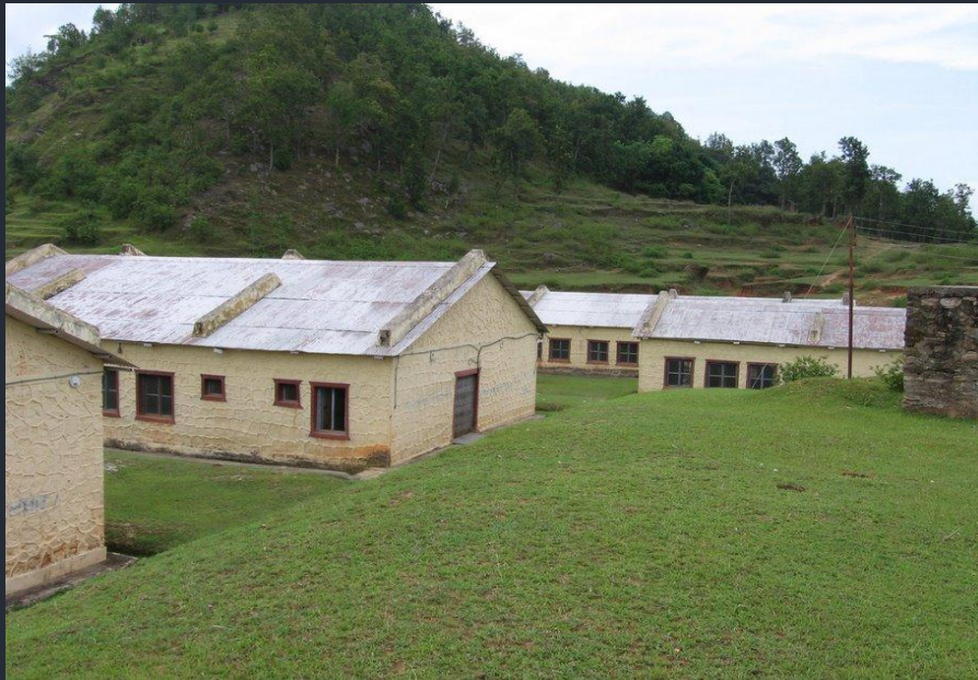
Bayalpata Hospital that Nyaya is renovating
